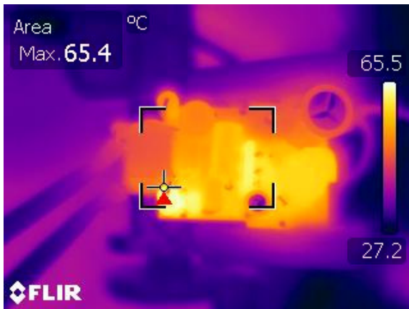
Figure 23 – With TRIAC Dimmer Connected. V_{IN} = 120 \text{ VAC} , 60 Hz, 15 V LED. Load at Full Conduction. R4 was Hottest Device.
